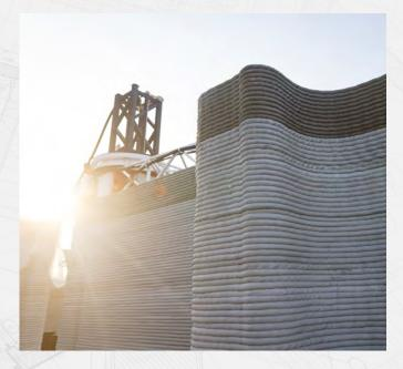
3D construction printing is another rapid innovative construction method, which leverages 3D printing technology to build affordable housing, including semi-detached and detached homes. It is also a more cost-effective housing solution than traditional builds.<sup>102</sup> Australia needs to incentivise the wide uptake of this efficient construction technology to address the housing crisis.
